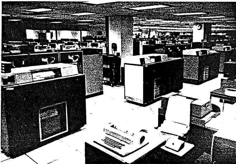
Figure 2.2 Typical Computer Installation within Industrial Facilities (Ref. 22)
